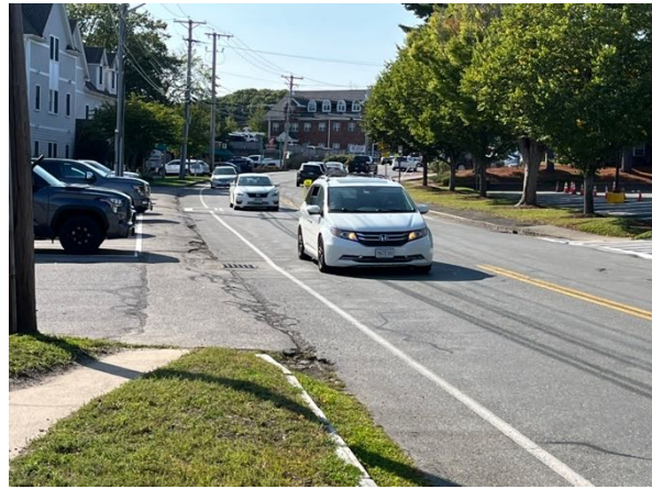
Detail of discontinuous pedestrian route, lack of delineation between road and parking area
