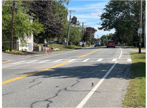
Eastbound at KinderCare: shoulder is less than 4 feet wide and driveway paving overlaps making shoulder uneven
