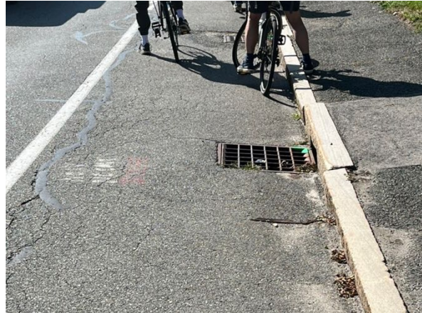
Storm drain grate in shoulder on Low Street at Port Plaza, reduces effective bike lane width to about 4 feet.
