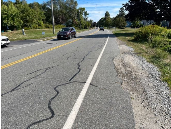
Eastbound opposite Tennis Club: deteriorating pavement reduces effective shoulder width to about 2 feet
