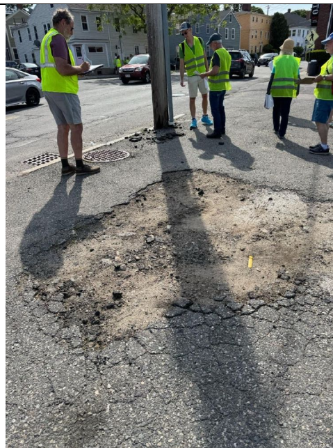
Sidewalk at oil company
